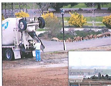
Figure 1. Chute washwater being dumped on the ground
